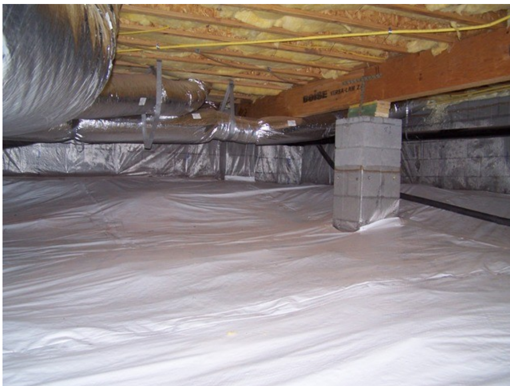
Figure 20. Flagstaff finished floor-insulated closed crawl space.
