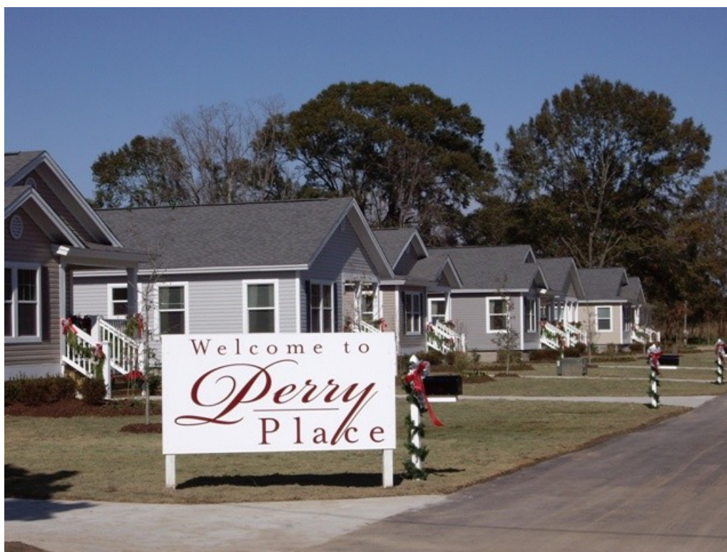
Figure 5. Baton Rouge street view.
