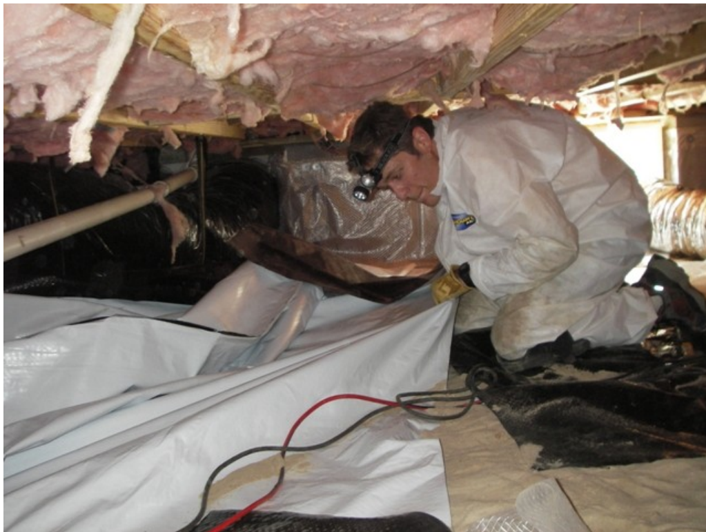
Figure 8. Baton Rouge liner system installation.
