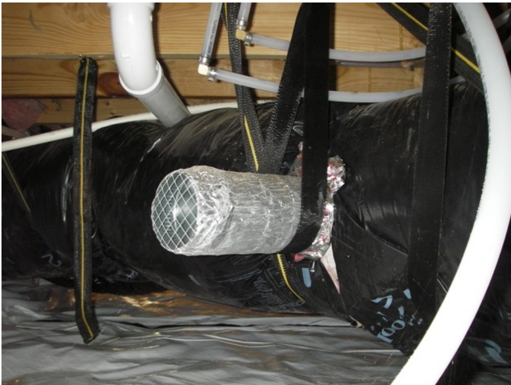
Figure 11. Baton Rouge closed crawl space drying mechanism.
