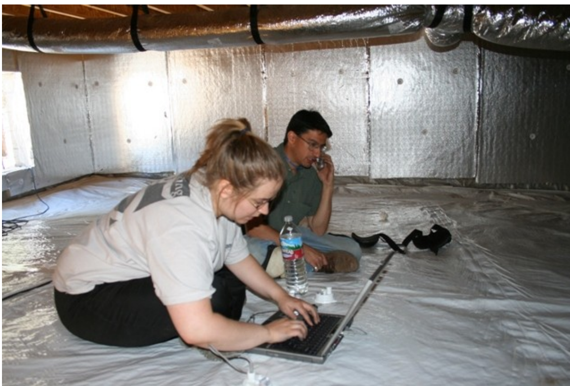
Figure 21. Flagstaff finished wall-insulated closed crawl space (doubling as an Advanced Energy field office).
