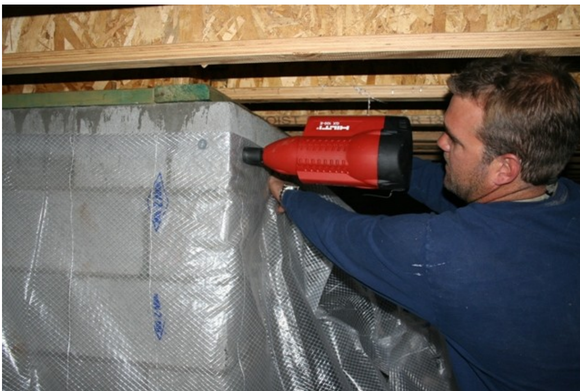
Figure 19. Flagstaff wall liner installation.
