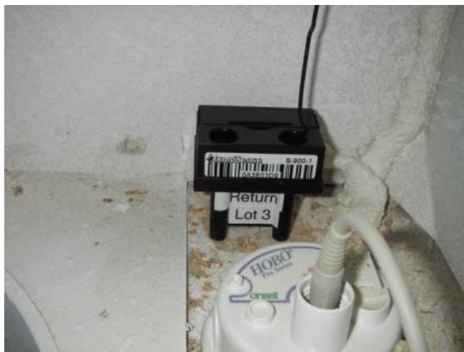
Figure 23. HVAC return OmniSense sensor mounting with adjacent HOBO logger.
