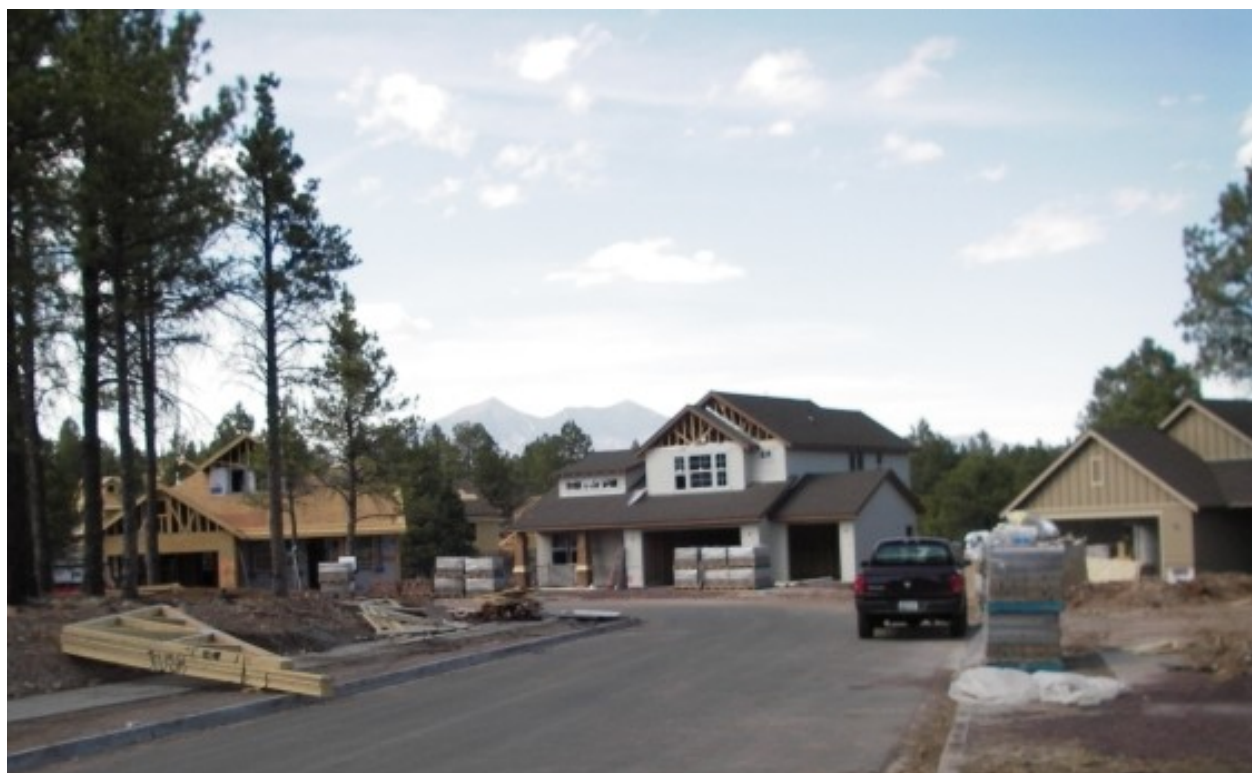
Figure 16. Flagstaff site during construction.
