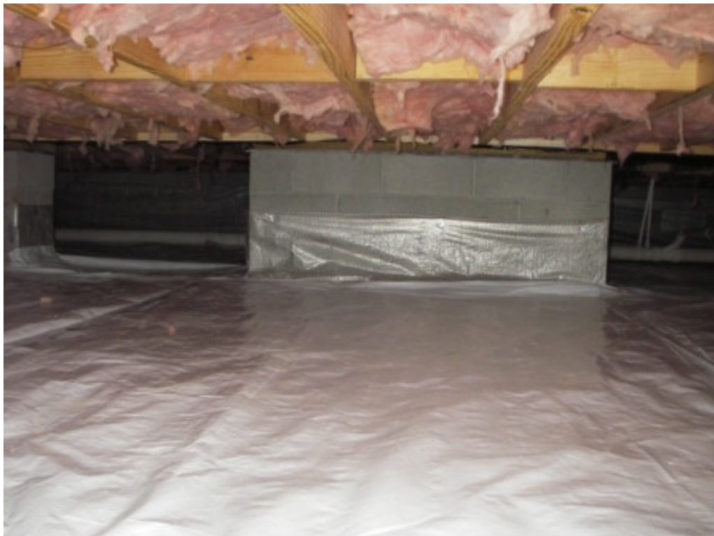
Figure 9. Baton Rouge finished floor-insulated closed crawl space.
